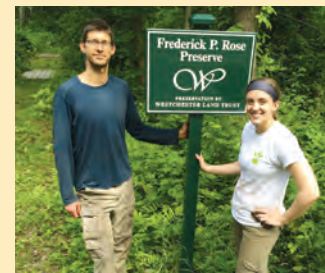
Sara and Tate recently constructed a new wooden bog bridge at the Frederick P. Rose Preserve (Lewisboro).
